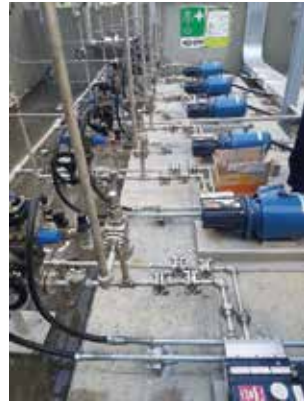
Aqueous Ammonia Supply Pump
